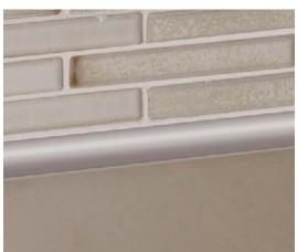
RONDEC-STEP edging profile applied to the sink rail. RONDEC bullnose profile and large radius sink corners used to produce the tiled-under sink. DILEX-AHK cove-shaped profile used to create a smooth, easy-to-clean transition between the countertop and backsplash.
