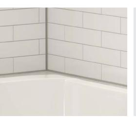
JOLLY profile and matching corners used to finish the tile edges on the walls and tub surround. DILEX-EKE eliminates the need for caulking, and creates smooth wall/countertop, wall/tub, and wall/floor transitions.
