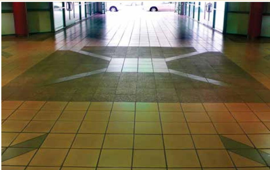
*This tiled floor on the ground-level public/retail areas of Phoenix Plaza in Oakland, Calif., was installed in 1989. It was set over DITRA uncoupling membrane, installed on post-tensioned concrete over a parking garage. It has endured frequent use – including the 7.1 Loma Prieta earthquake – and is still in excellent condition today.*
