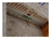
Embed the profile at the top of the niche. Pull the wire tape tab down through the thin-set mortar and slot in the profile. Be sure the wire can move freely. Clean away all thin-set mortar from the tape, wires, and channel.
