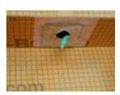
Remove the paper backing on the KERDI patch and adhere it to the same location as it was tested. Carefully smooth the KERDI from back to front, so there are no bumps or wrinkles.
