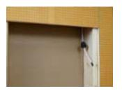
Once the cut piece of KERDI-BOARD or solid backing has been removed, locate the previously run LIPROTEC-CW connection cable. Please refer to the KERDI-BOARD-SNLT Planning Guide for determining and configuring the required length of the LIPROTEC-CW connection cable for your application.
