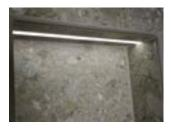
Fill in any gaps at the end of the LED above the tiles with grout or caulk.
