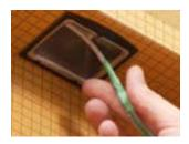
Add **masking tape** around the connector on the LIPROTEC-CW connection cable below the cable gland. The tape protects the connector from being fouled by thin-set mortar. Use extra masking tape to create a tab to pull the wire out of the box during installation.
