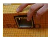
Insert the stainless steel connection box into the plastic cavity at the top of the KERDI-BOARD-SNLT niche. Hold in place as you locate and grab the cable gland end of the LIPROTEC-CW connection cable.
