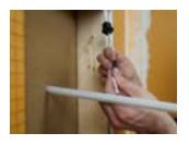
Test the LED function by connecting the waterproof plugs together (LED connector to end of LIPROTEC-CW cable). Check all connections are complete and correct at the LED power supply (LIPROTEC-ECX driver). Turn on the power and confirm the LED will illuminate by using the wall switch. Note: DO NOT test the LED function by connecting the LIPROTEC-CW cable directly to 120V power. This will damage the LED strip light, could result in electrical shock, and will void the warranty.
