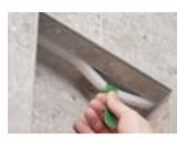
Allow thin-set mortar to cure and apply grout. If you do test the fit of the LED strip into the mounting profile, it must be removed prior to grouting. A tab can be made with masking tape to facilitate removal. It is important to remove the LED strip from the profile prior to grouting to avoid damage.
