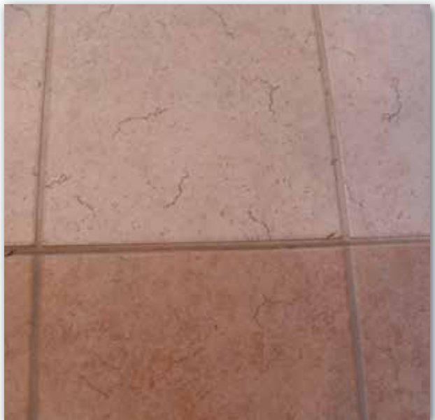
Properly-placed movement joints - here filled with DILEX movement joint profiles - help ensure the floor stays crack-free and are virtually indistinguishable from grout joints in the floor.
