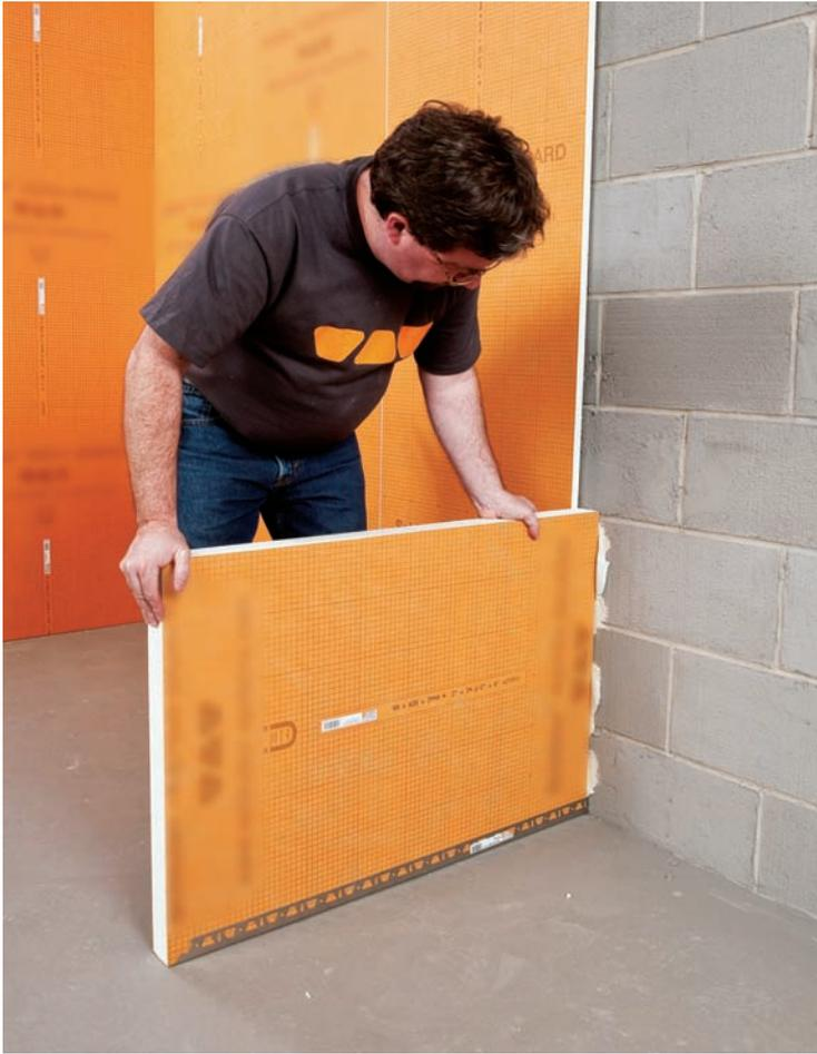
Waterproof polystyrene building panels can be used to construct tile-ready elements such as partition walls without any wood or metal framing.
