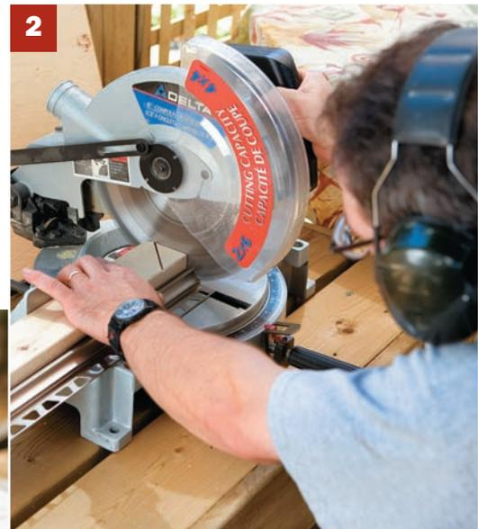
**2.** The profile pieces can be easily cut with a non-ferrous metal blade in a chopsaw, or by hand with a simple hacksaw. (For more information on the Schluter edging, call 800-472-4588 or go to [www.schluter.com](http://www.schluter.com))
