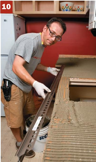
**10.** Lay the edging pieces in position over the mortar, pressing them in so their perforated flanges are grabbed by the mortar
