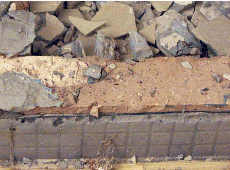
*Top Left: This one-and-a-half-year-old shower had a glass mat backerboard nailed to the top and back of the concrete curb through the shower pan liner. The original complaint was that the tile fell off the inside of the curb. Further investigation revealed additional leaks at the pan liner corners, which had been cut and not seamed properly.*
